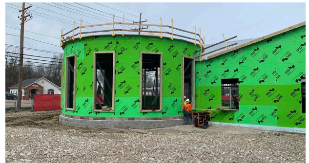
South addition exterior sheathing
