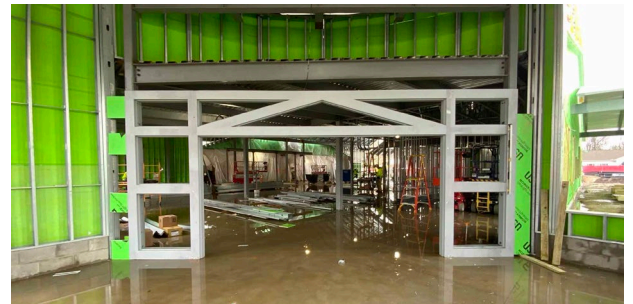
Installation of the Greenhouse doorframe in the children's area
