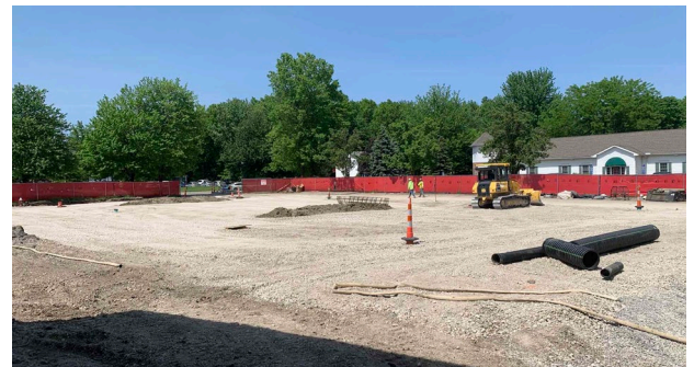
Completion of Northeast retention system
