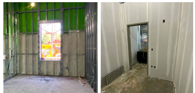
Spray foam and drywall for the South addition
