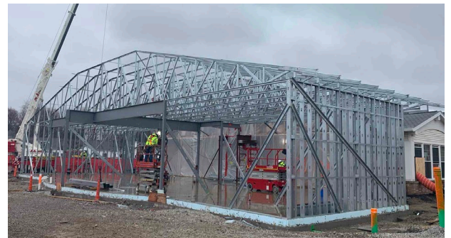
North addition truss installation
